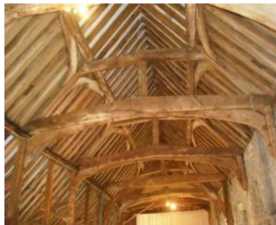
Left: The Long Gallery with its first floor, timber framed open gallery (now covered with cloth blinds) Right: The splendid roof trusses of the gallery, formerly subdivided into several grand chambers, accessed from the long corridor on the left.
